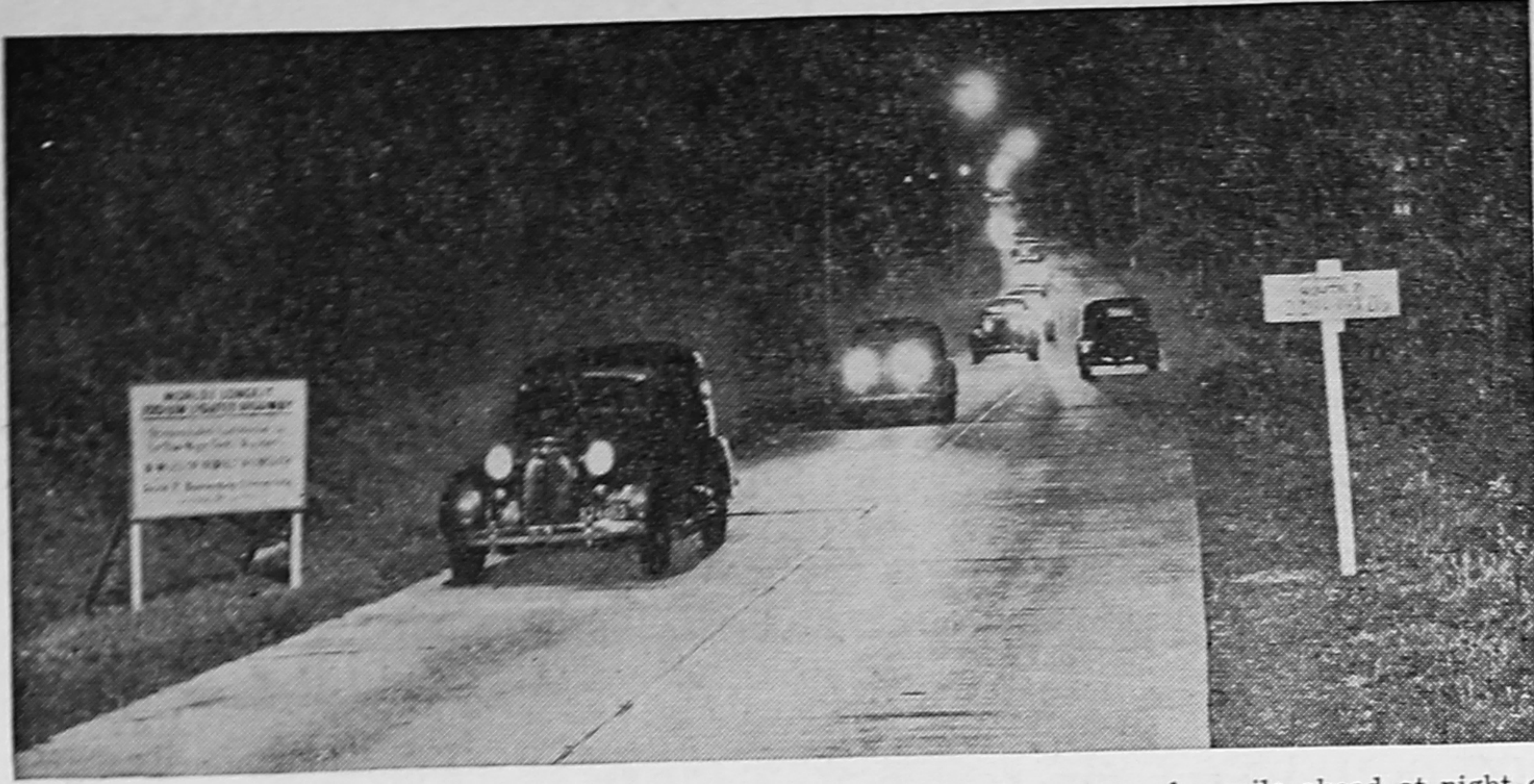
A motorist can see a pedestrian a half mile ahead and a car three-quarters of a mile ahead at night on the illuminated highway between Schenectady and Duaneburg, N. Y. The 18-mile stretch of road is lighted with 390 yellow sodium lights spaced 250 feet apart by engineers of the General Electric company and the American Road Builders' association.
