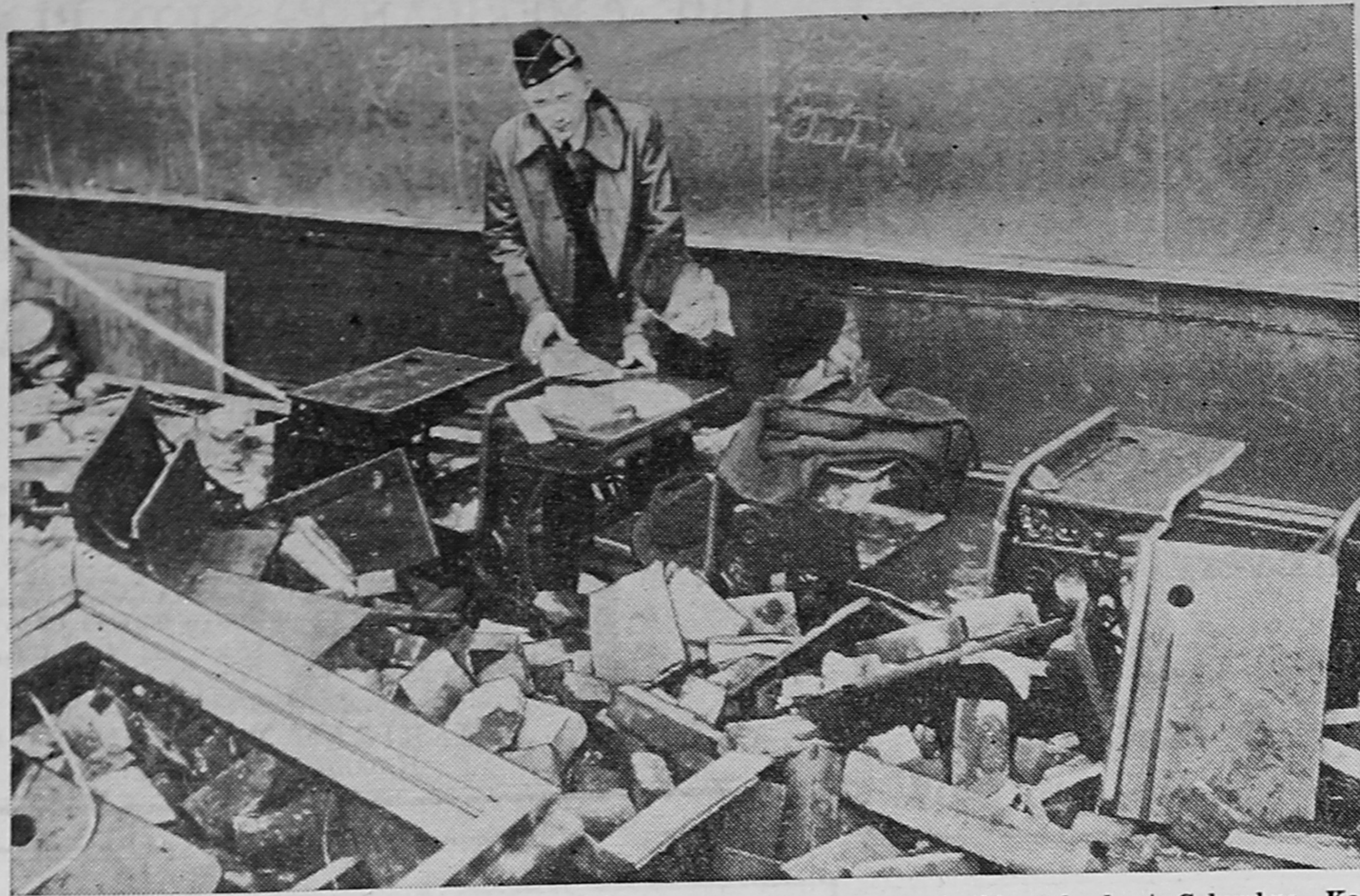
A tornado which swept destruction from Arkansas to Illinois wrecked this school at Columbus, Kan. Luckily none of the pupils were in their rooms when the twister hit. This picture shows a member of the American Legion with his little son as they recovered his things from a desk in the wrecked school room.
