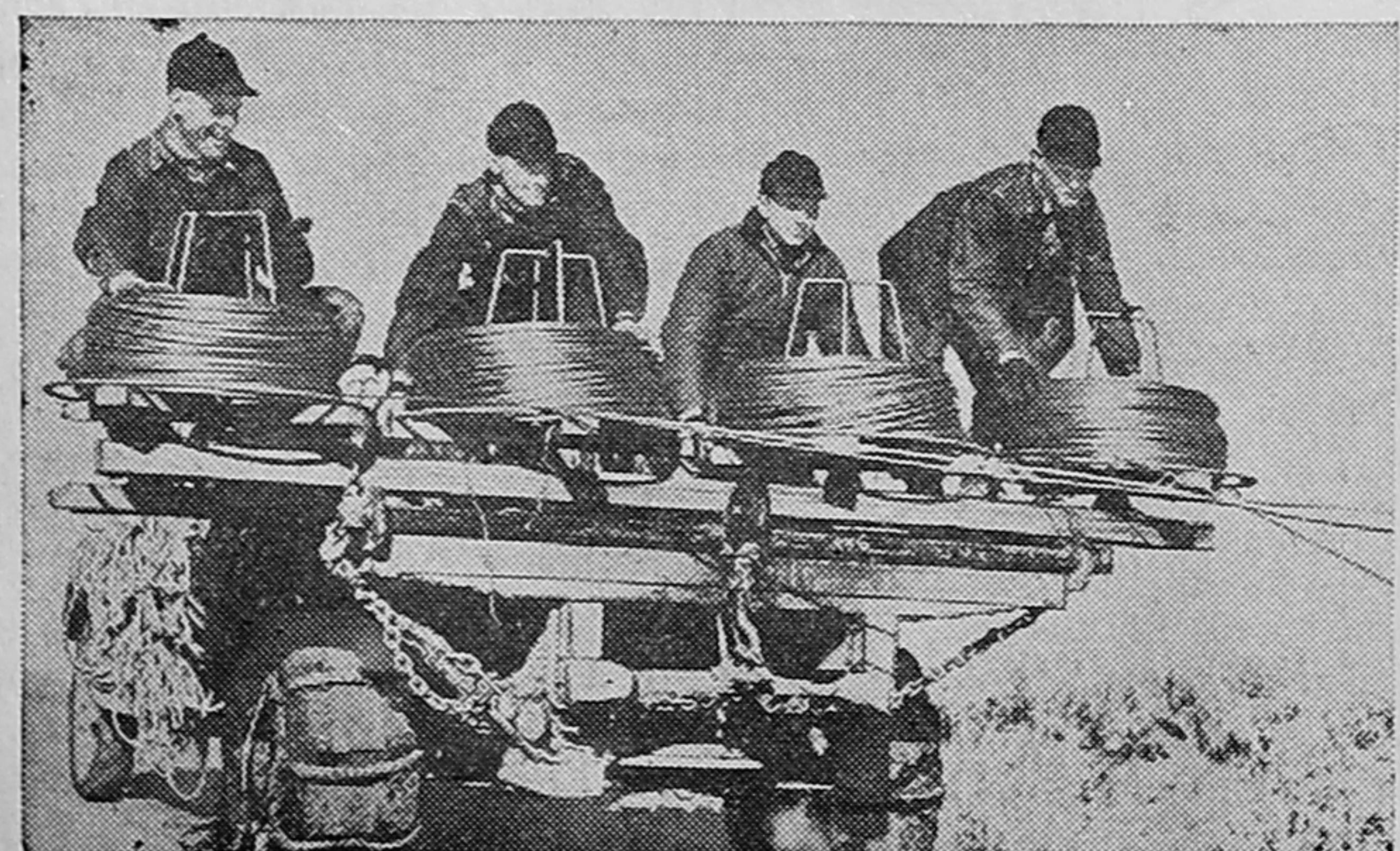
Stringing four lines of aluminum cable at once near Horton, Kan. REA projects have required 115,000 miles of this cable.
