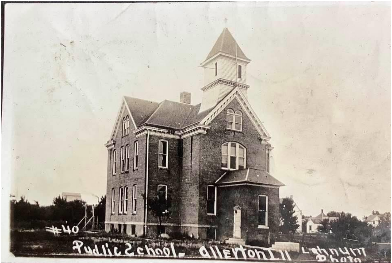
The Allerton public school was built by Frank Gray of Danville in the fall of 1893.
